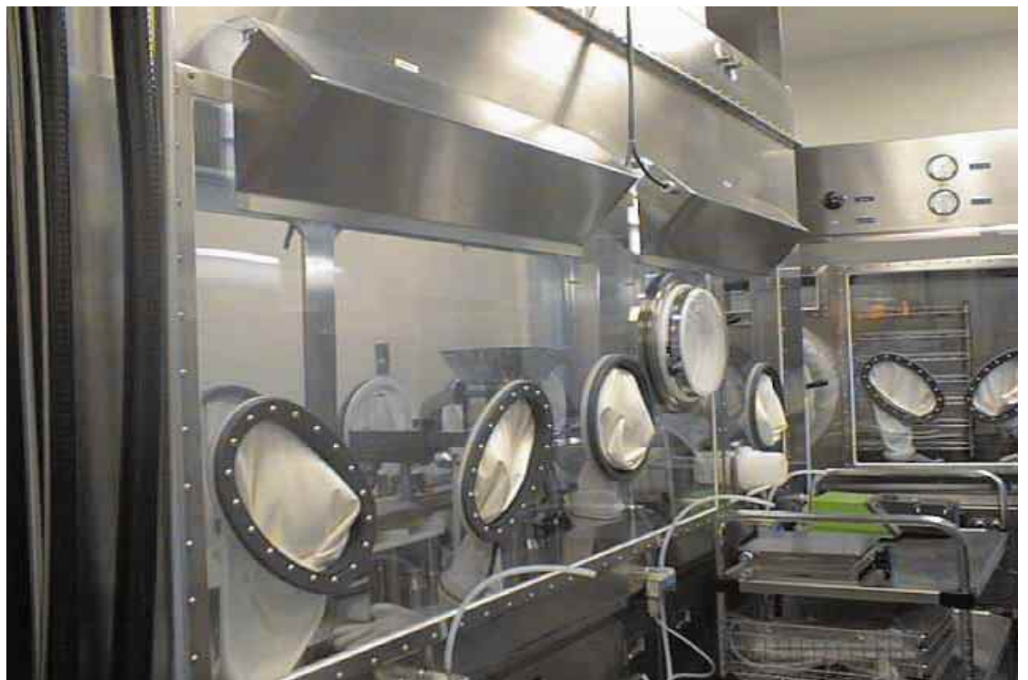
Figure 3b: Carlisle Barrier Filling Isolator (Rear view)
